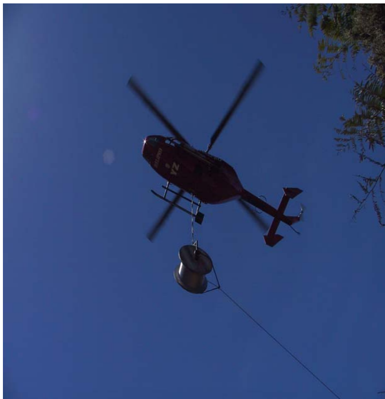
A Helipro BK 117 stringing a cable
